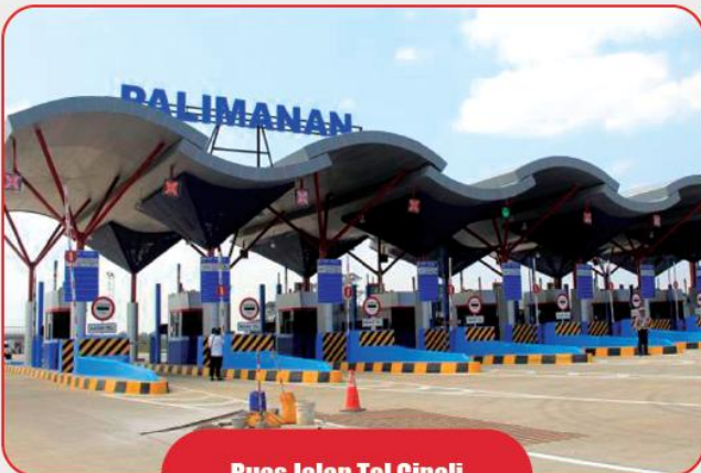
Ruas Jalan Tol Cipali
